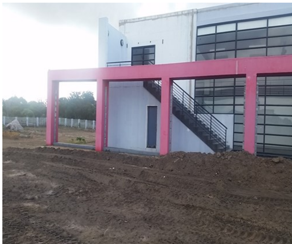
Parking lot under construction
