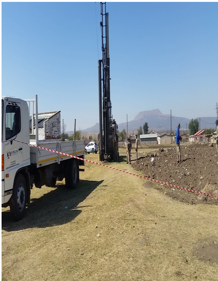
Drilling machine owned by the company
