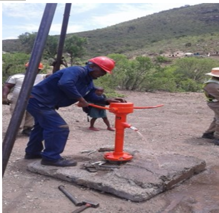
Repaired T7 Hand pump
