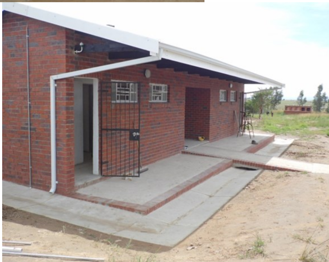
New sanitary facilities
