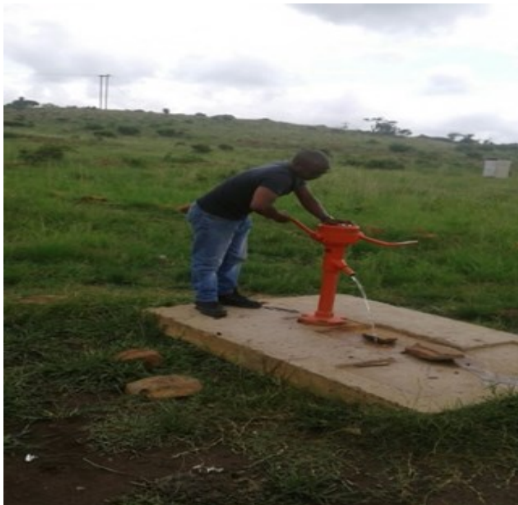
Restoration of the damaged/malfunctioned T7 Hand pump
